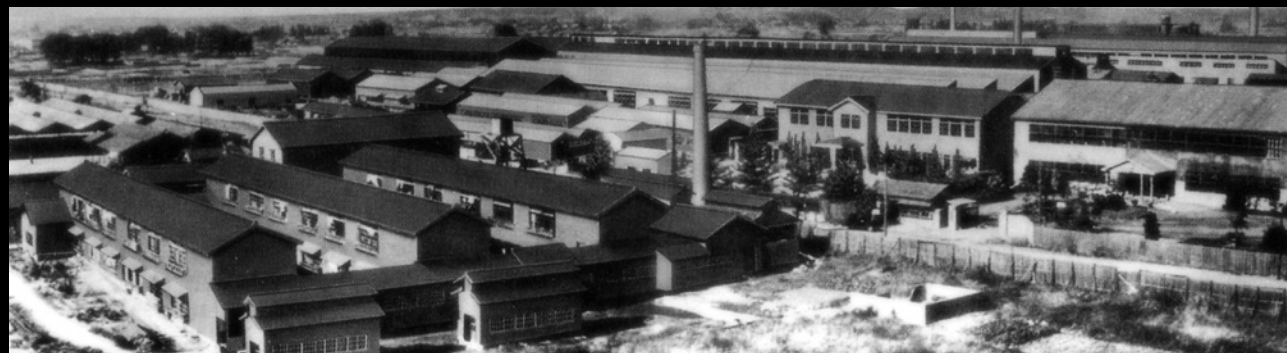
Kariya plant in 1952
